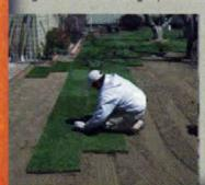
Avoid gaps or overlaps. Stagger the joints in each row in a brick-like fashion (use a sharp knife to trim corners). A knife with a serrated edge works very well.
